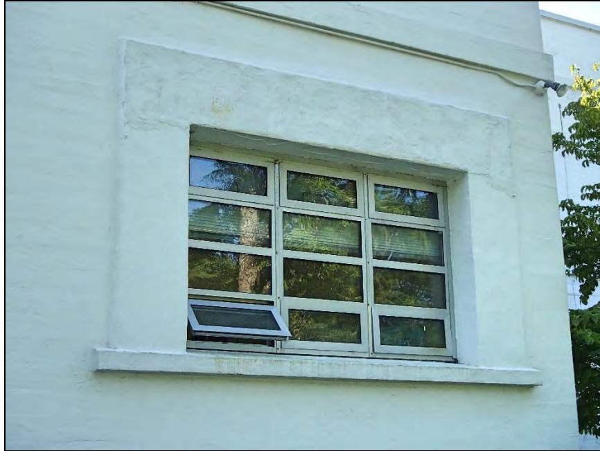
8: NCSCF, window detail
