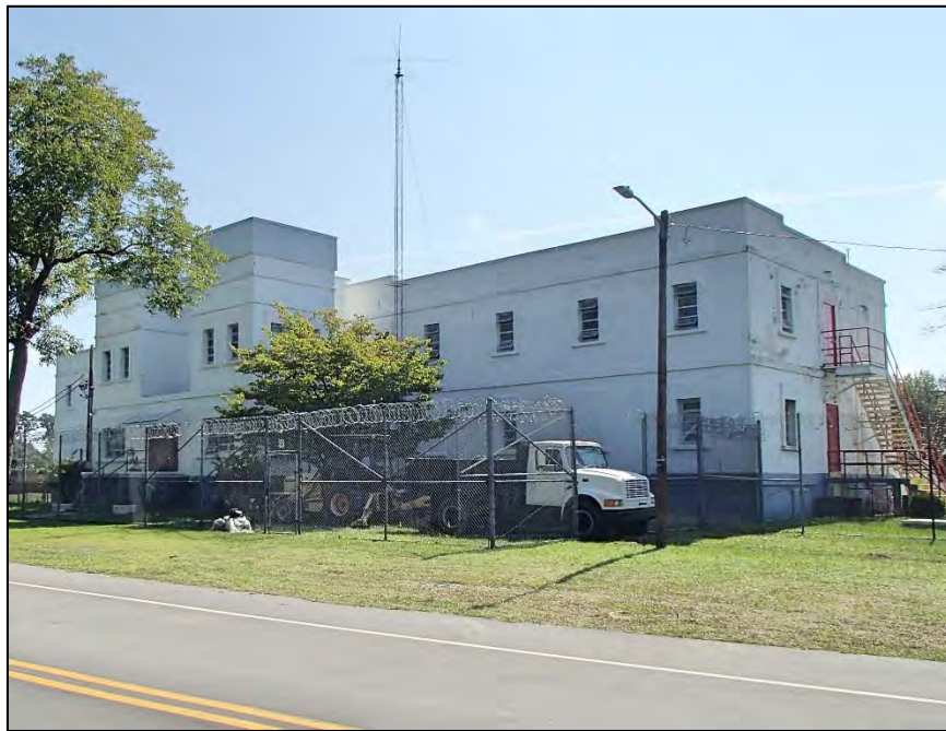
7: NCSCF, west and south elevations
