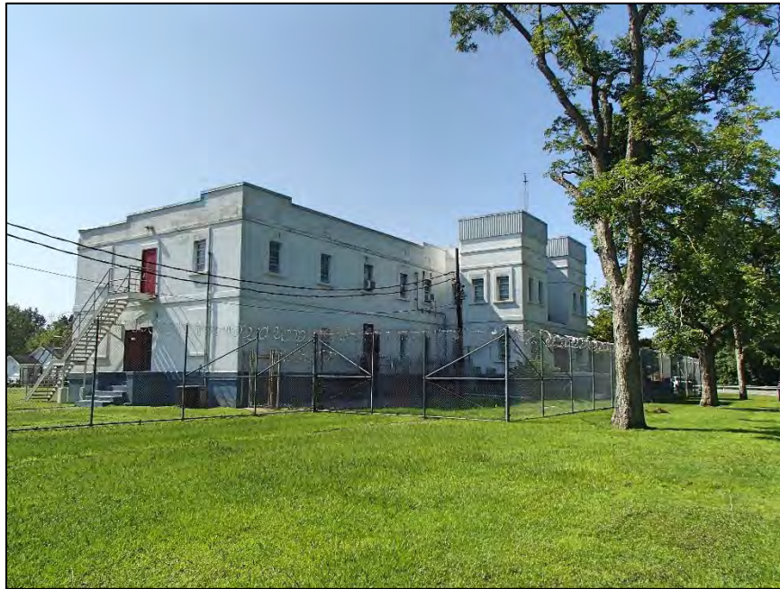
4: NCSCF west and north elevations
