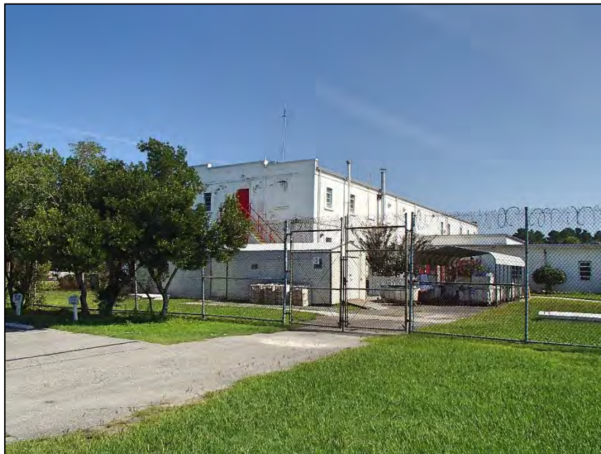
10: NCSCF, south and east elevation
