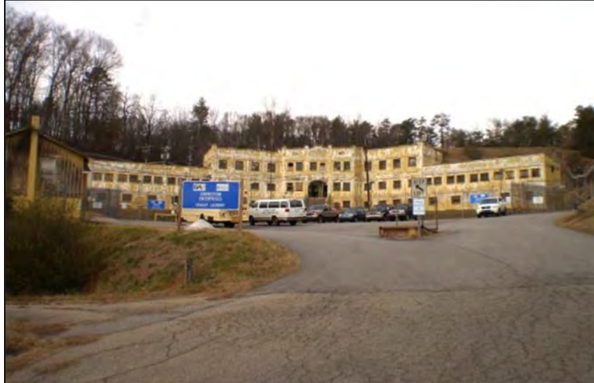
20: former Craggy Mountain Prison, photo from A Thousand Country Roads , accessed via https://www.athousandcountryroads.com/2017/03/im-stuck-in-craggy-prison.html
