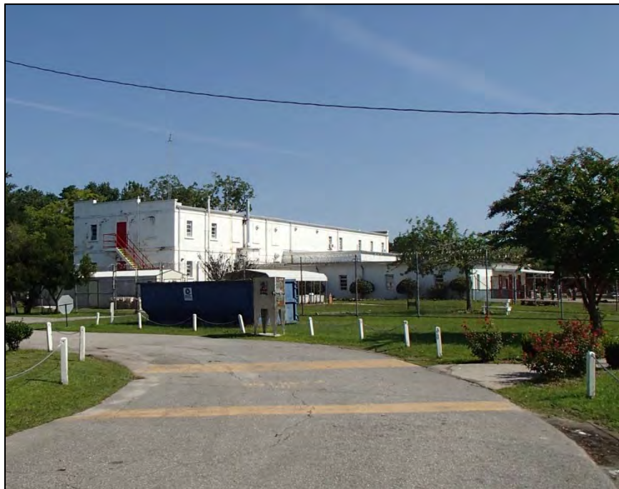
12: NCSCF, southeast corner
